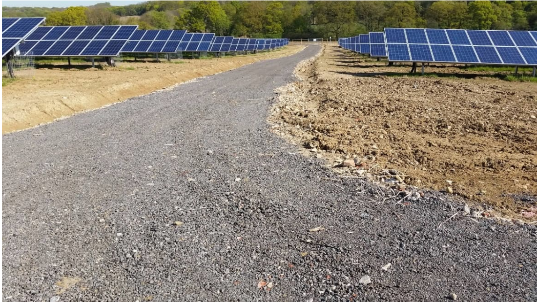
Plate 2-10: Typical crushed stone access track laid on hardcore and geotextile (photo during construction phase and prior to landscaping)
